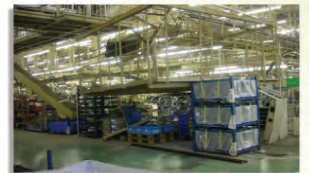
Japan's devastating earthquake damaged Nissan's Iwaki engine plant. The image shows fallen ducts and pipes.
