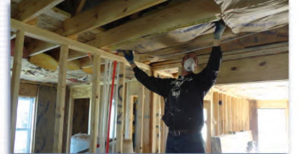
Toyota's continuous improvement techniques helped the St. Bernard Project streamline home rebuilding efforts in Louisiana.
