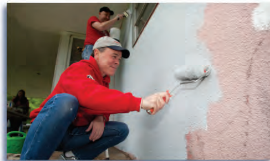
Honda, Rebuilding Together Central Ohio
